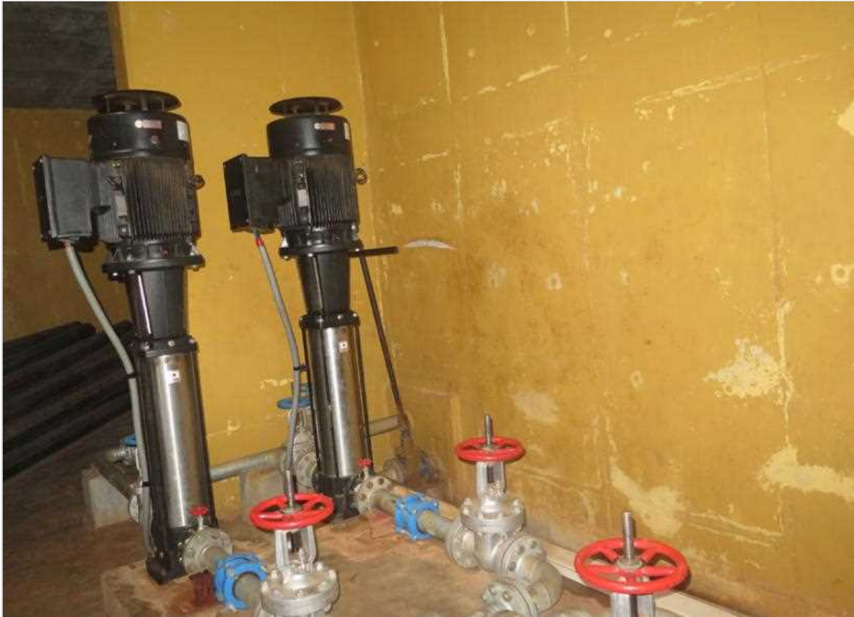
Water pumps in Rwakibogo pumping house. The pumps feed three sectors in Rwamagana districts.
